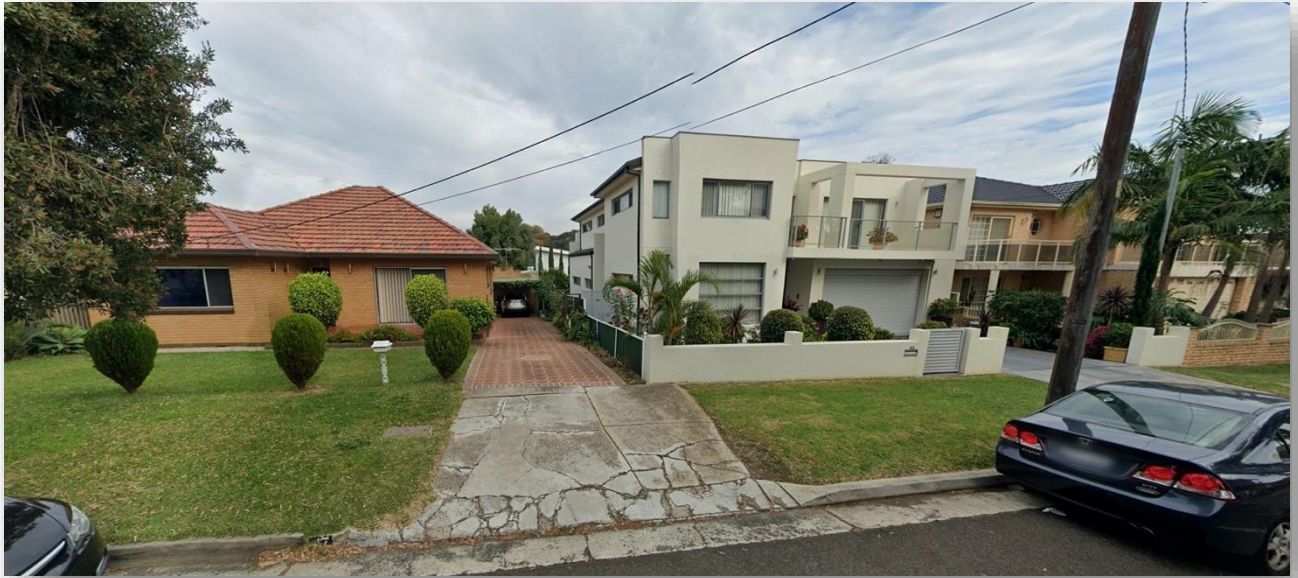
Figure 15: Examples of modern infill development in Emily St amongst older style development typical of locality. (Source: Google Maps: Image capture May 2019©2020 Google)
